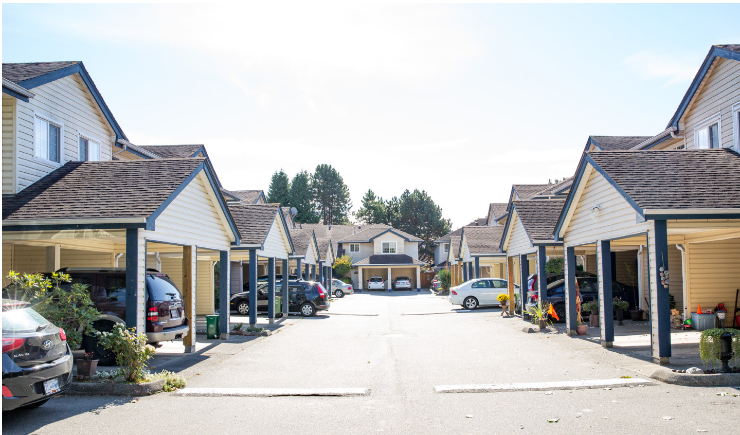
Example of a Housing Co-operative in Richmond
